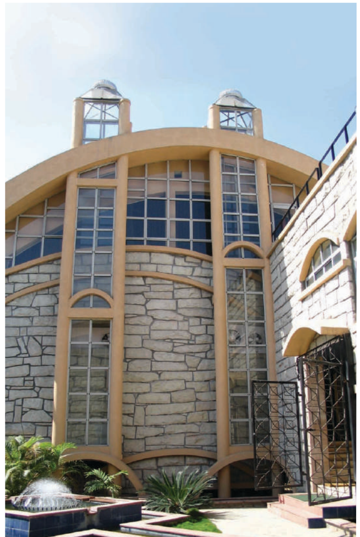
A 'green' building
